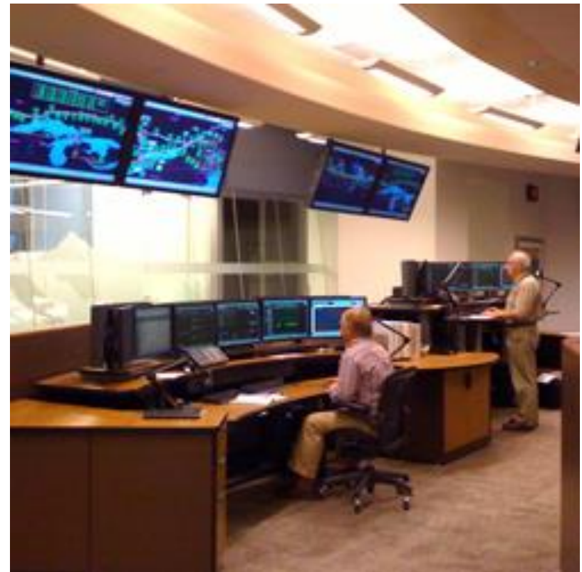
Control center in Calgary Alberta
