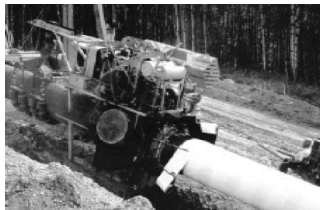
Figure 3: Field applied polyethylene tape coating
