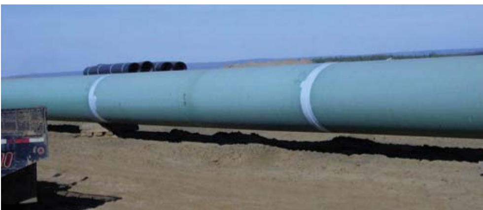
Figure 2: FBE Coated Pipe
